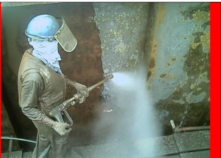
Pictures showing Ultra High-Pressure Hydro-blasting to remove completely all remaining original coating system. Surface cleanliness to NACE WJ2. Original surface profile to SA 2 ½ restored. Date of work commencement 15 th March 2002
